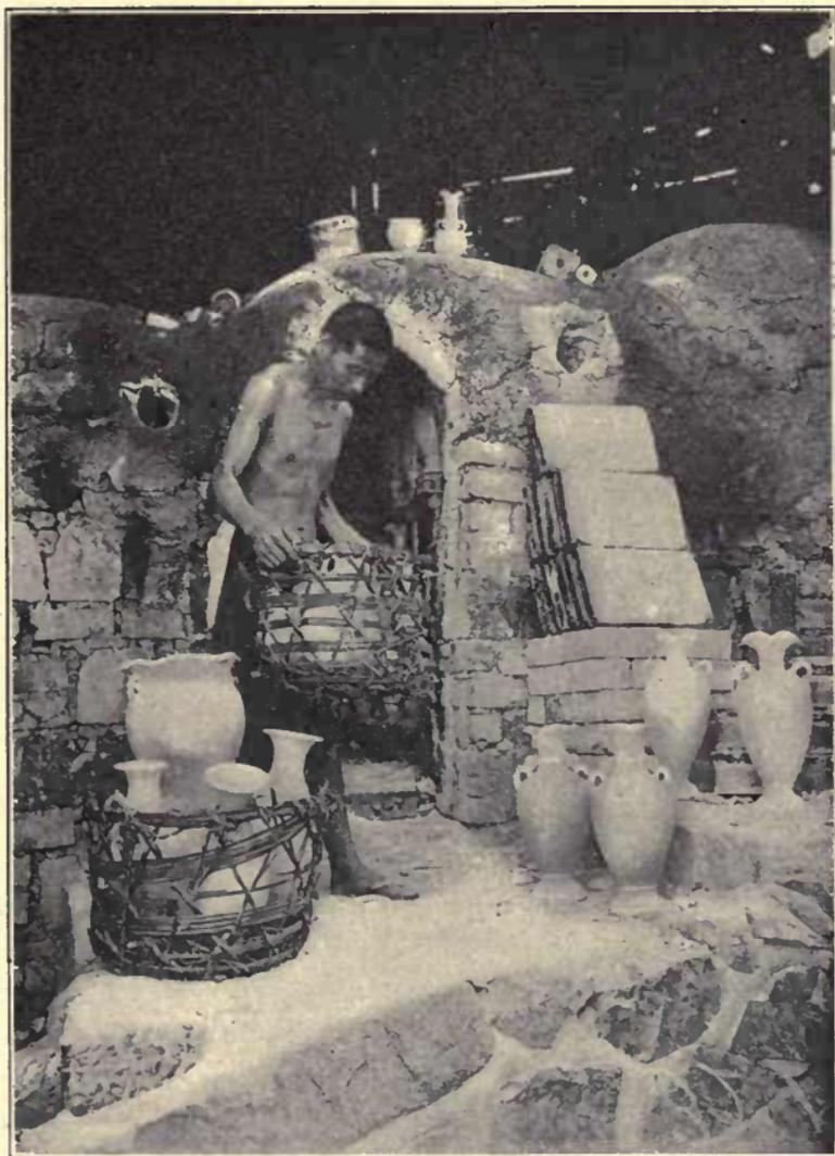
*Removing Pottery from Kiln at Kinkosan Works.*
